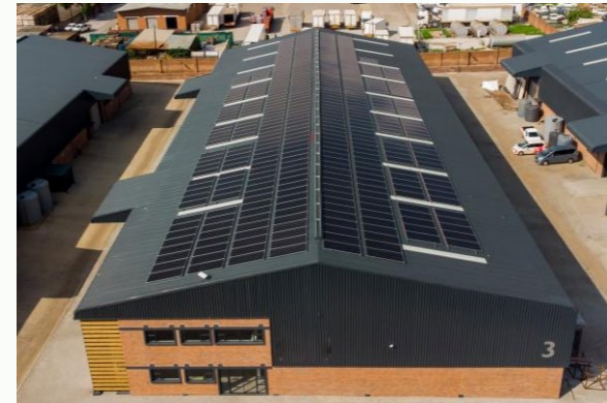
◀ 180 kW PV system of CNBM ZIM ▶
