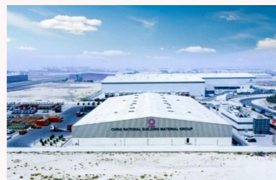
◀ Dubai overseas warehouse of CNBM ▶
