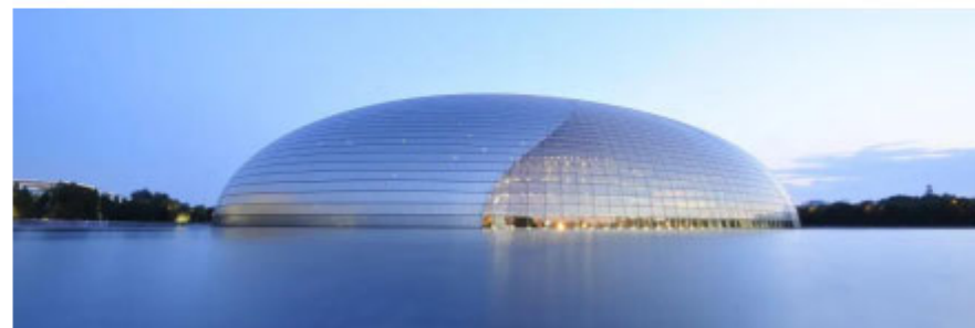
Dragon Brand Coating provides supporting products for the National Centre for the Performing Arts
