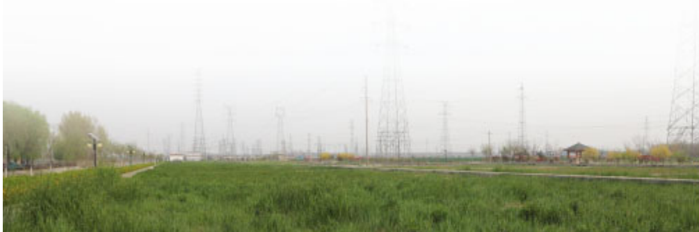
Taishan Gypsum Wentai Environmental Protection Tailwater Constructed Wetland
