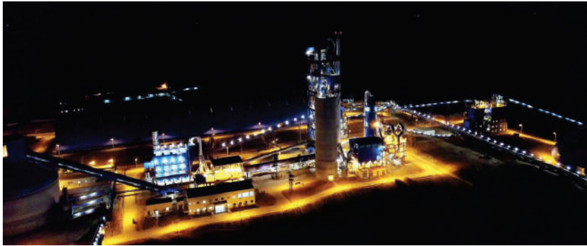
Night view of CNBM Zambia industrial park
