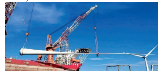
Lifting 123-meter wind turbine blades
